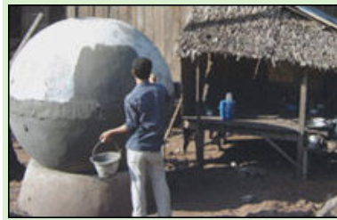
Applying Cement on the outside!
