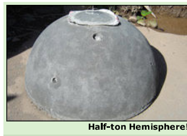
Ball Tank Building Activities!
